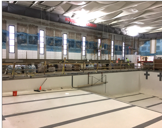
A view of the renovated pool area facing East looking across towards the spectator seating. New windows have been installed and ceramic wall tile work is being completed in the pool area. Below, wall tile is being installed in the girls locker room corridor.
